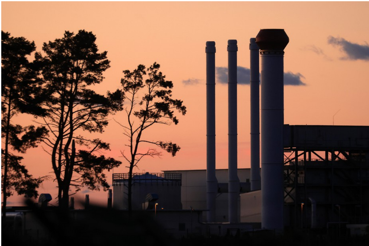
The gas-receiving compressor station in Lubmin, Germany (Krisztián Bócsi / Bloomberg / Getty)
